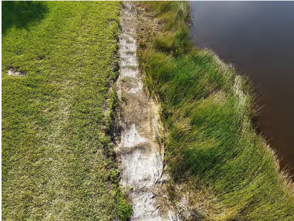
Lake 1 – Photo 3 2025 sod/fill repair.
