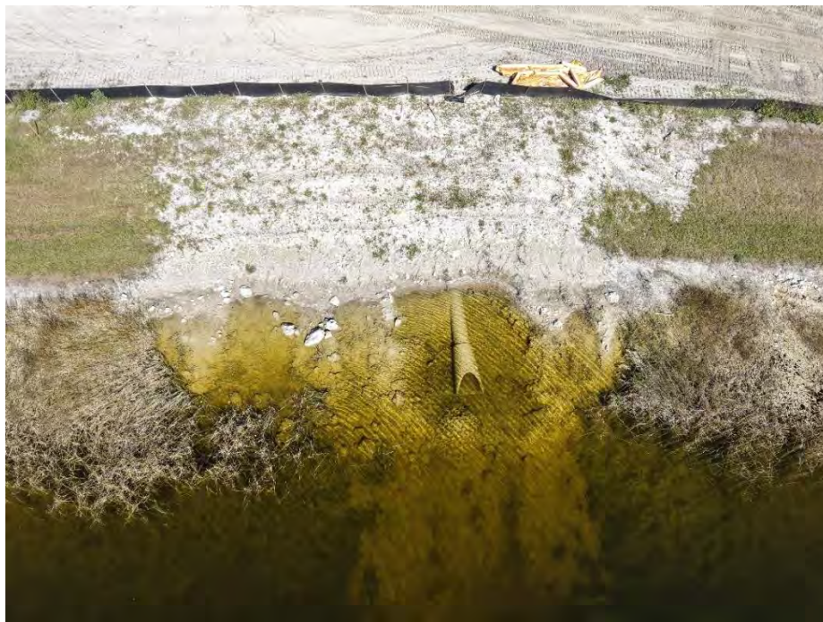
Lake 11 – Photo 62 Lake is adjacent to future residential construction. Lake bank disturbed by drainage installation. Additional sod required for stabilization.
