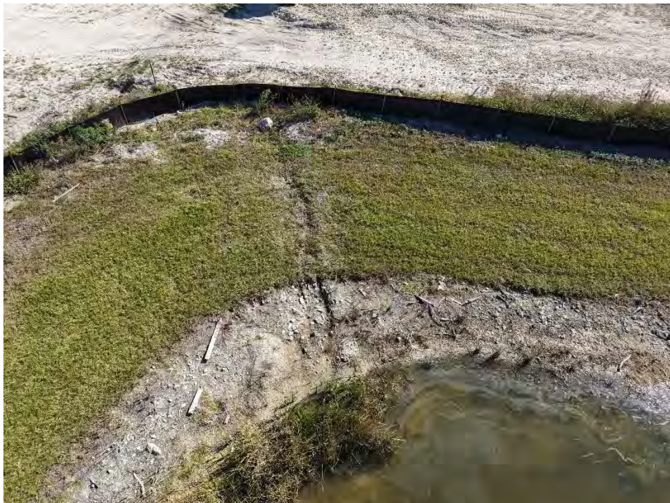
Lake 12 – Photo 66 Minor erosion on the lake slope.
