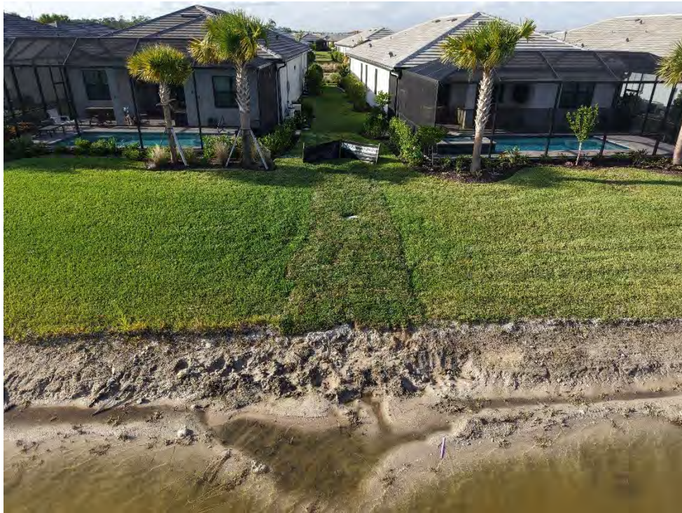
Lake 9 – Photo 51 2025 sod/fill repair.
