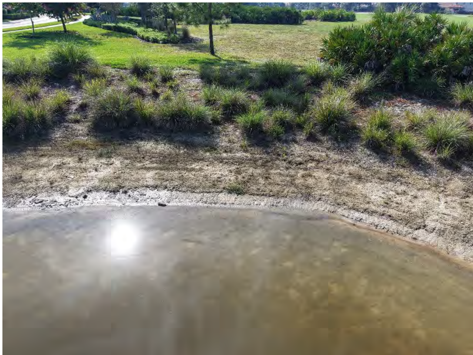
Lake 16 – Photo 78 Overall satisfactory sod is preventing erosion.
