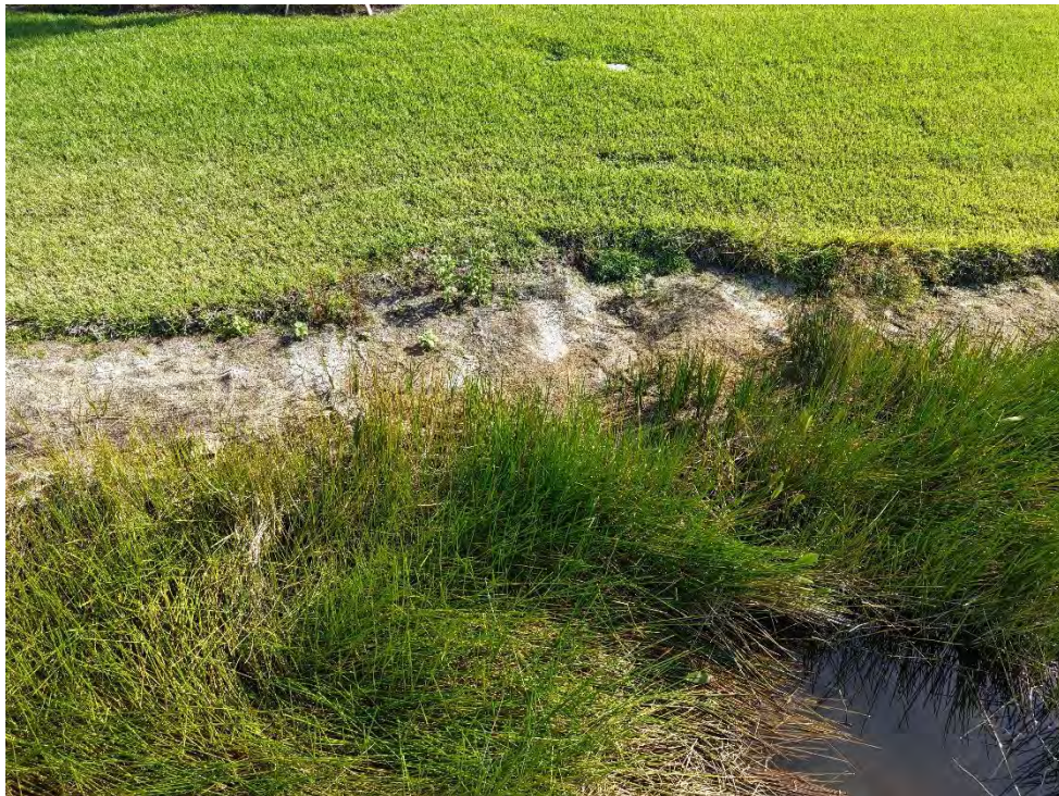
Lake 1 – Photo 4 Minor erosion on the lake bank slope.
